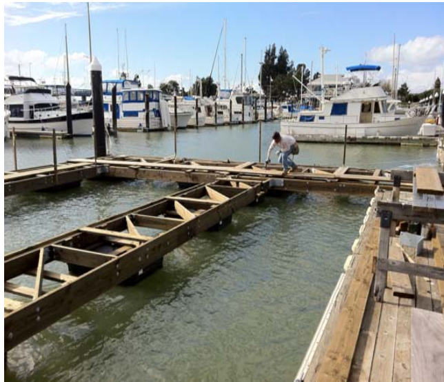
Repairing the "A" Dock
